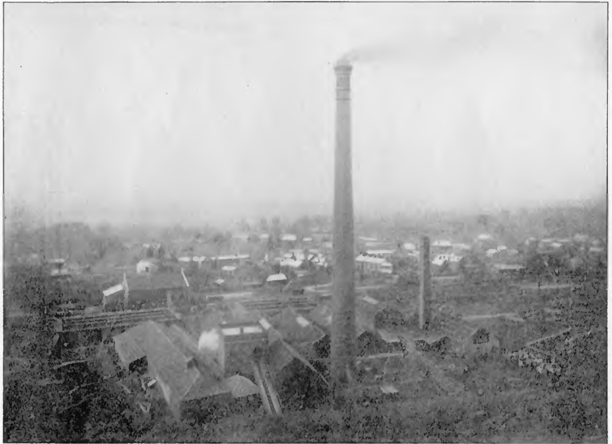
General View of the Stonehouse Brick and Tile Company's Works, Stonehouse
