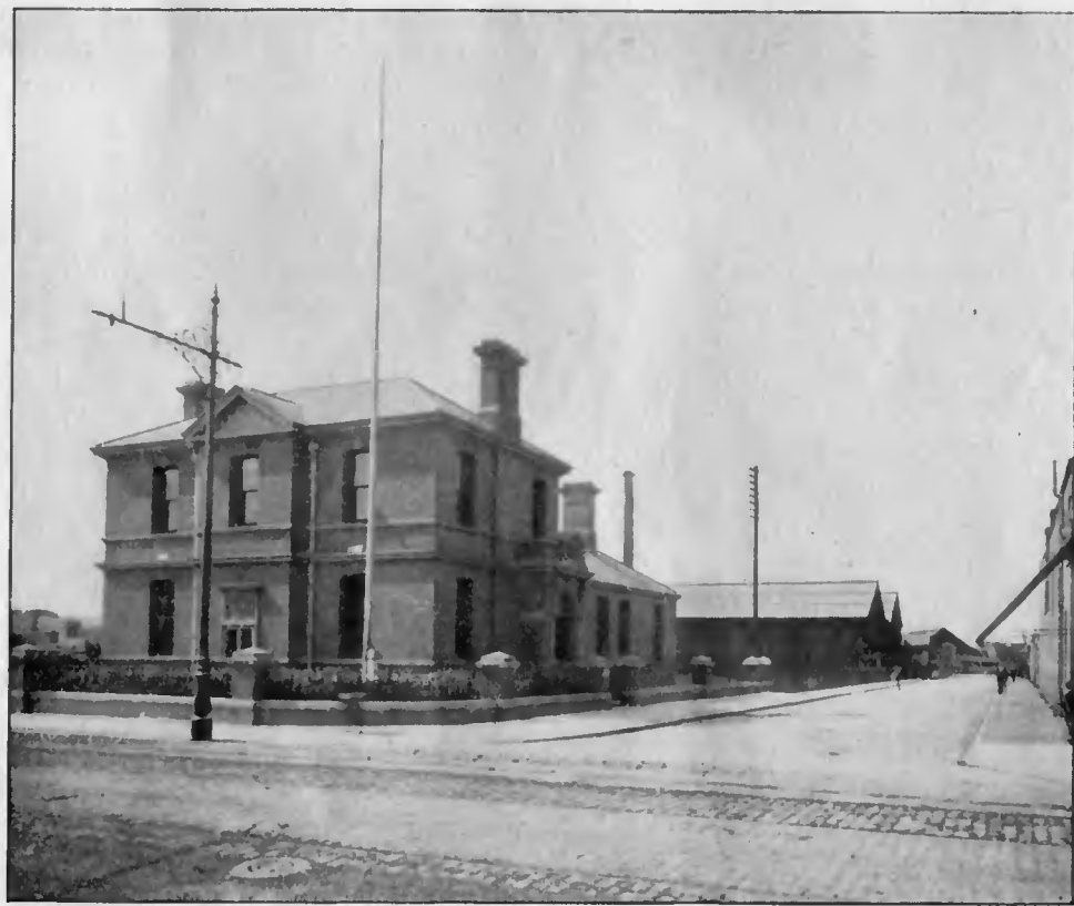
Offices and Principal Entry to the Works (Price, Walker & Co., Ltd.)
