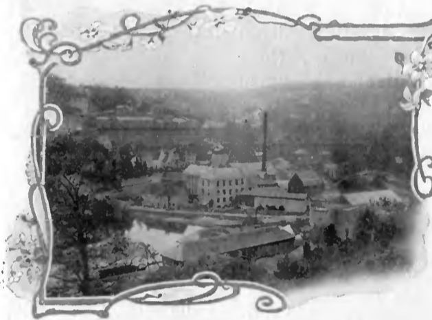
BRIMSCOMBE PORT MILLS. (P. C. Evans & Sons).
