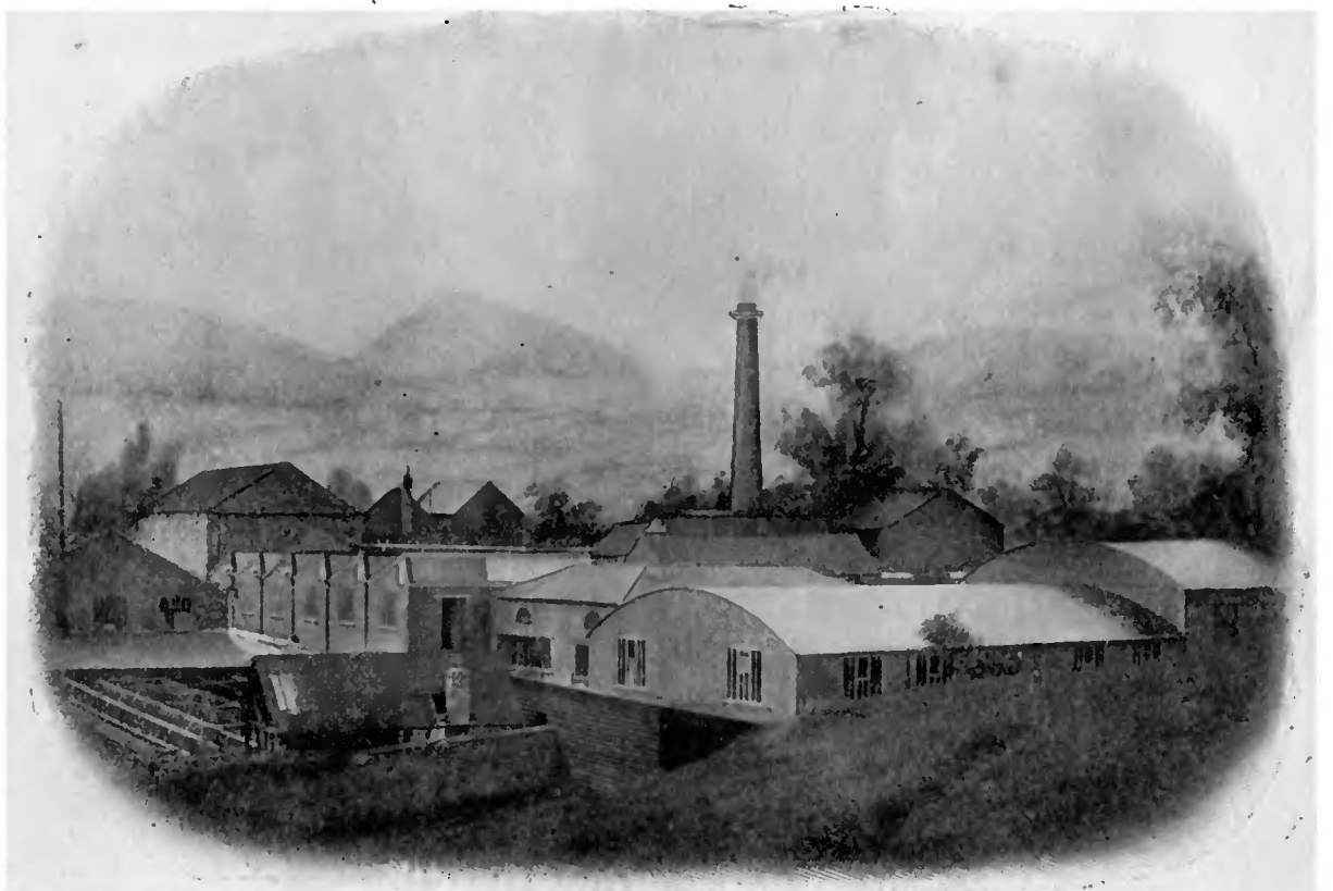
General View of John B. Champion and Sons' Works, Dursley
